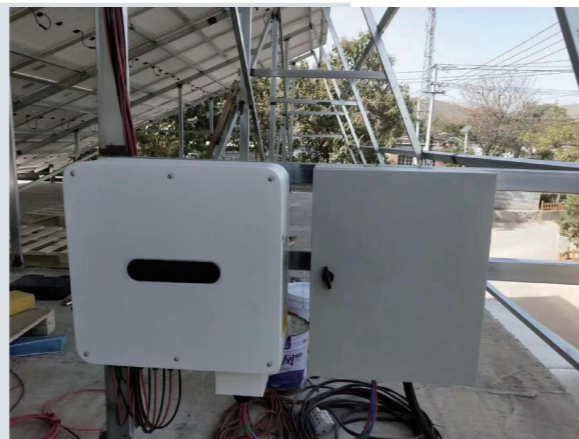
Residential PV Project in China
